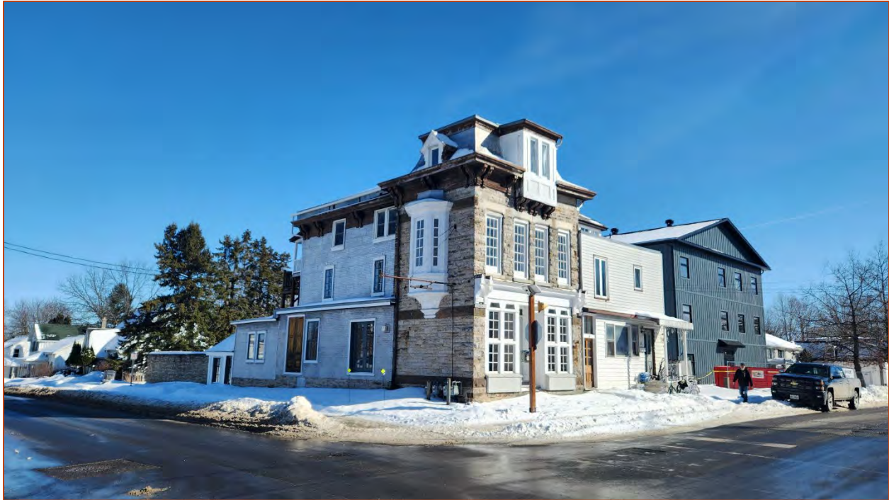
Photo 6. View east of two residential properties at the corner of Drummond Street East and Craig Street
