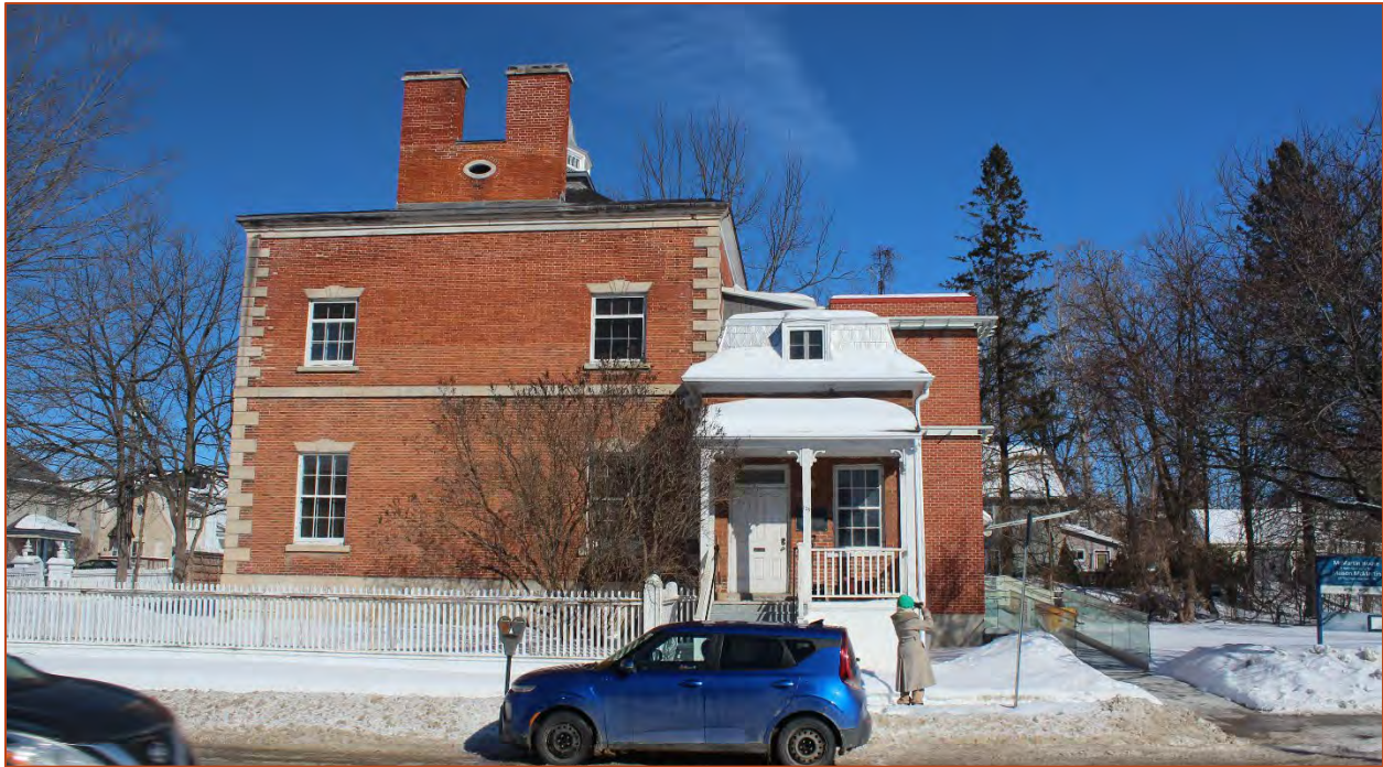
Photo 13. View northeast of the southwest facade of the McMartin House
