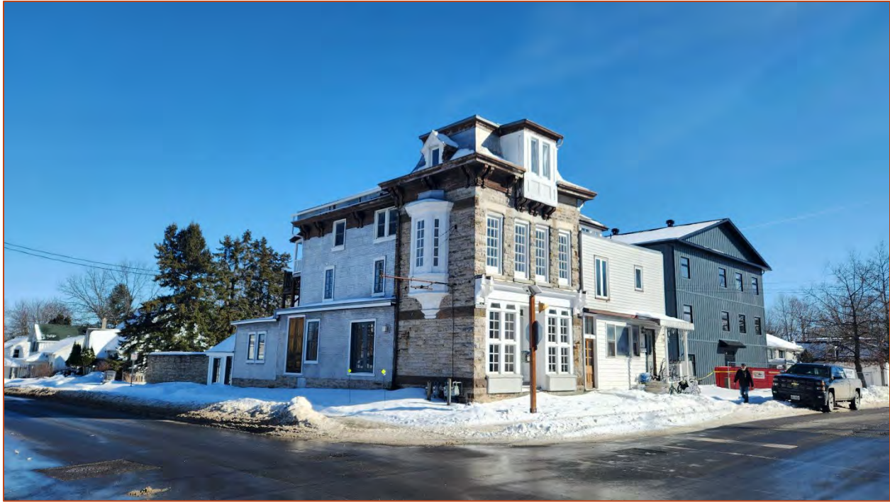
Photo 6. View east of two residential properties at the corner of Drummond Street East and Craig Street
