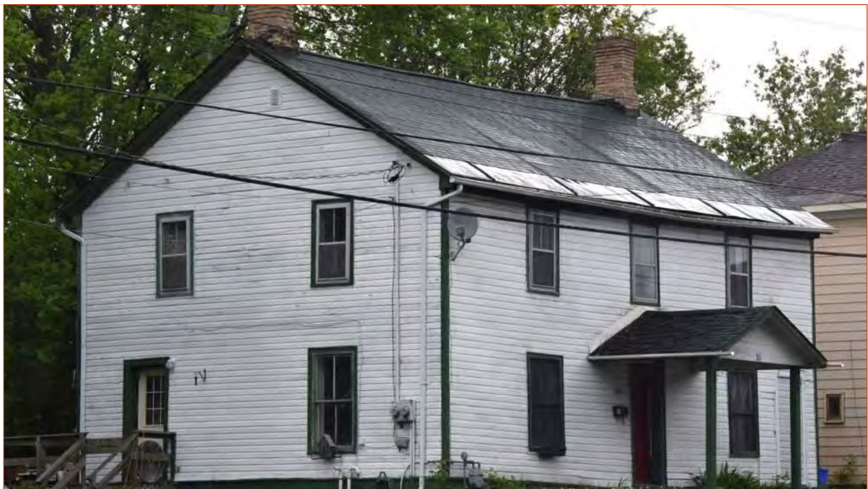
Figure 3. View of the original building on the site, date unknown 56
