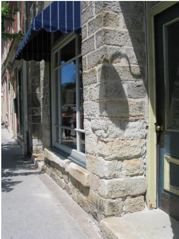
*Deterioration caused by salt and moisture requires stone replacement*
