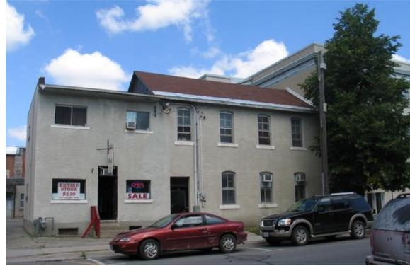
*Conversion to a new use does not require loss of original detail or character. Left – Perth Montessori School, 36-38 Foster Street, with new access at side of building. Right – side view of Ferrier Block, original building details lost under unsympathetic parge coat.*
